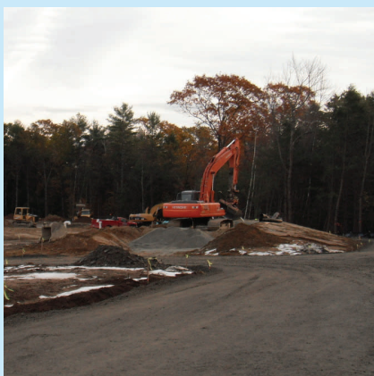
Commercial septic system installation in Brentwood
